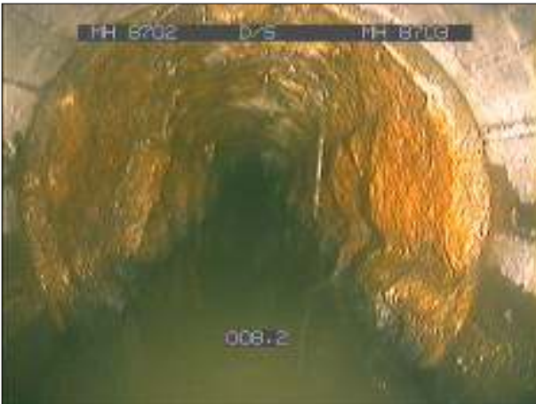
Photo: 247_5a, 00:00:48 8.2m, Sewer Material changes at this point, Cast iron
